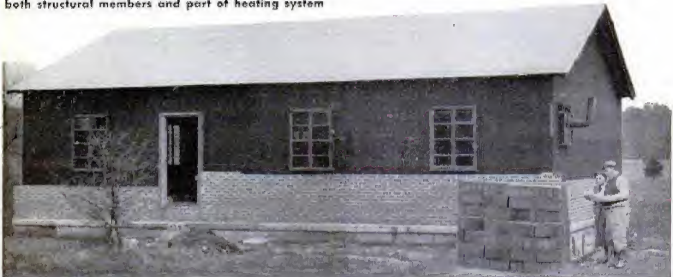
Wagner is covering the outside of his house with brick. The Celotex beneath the brick is fastened to the pipe framework. He estimates the cost at $5000
